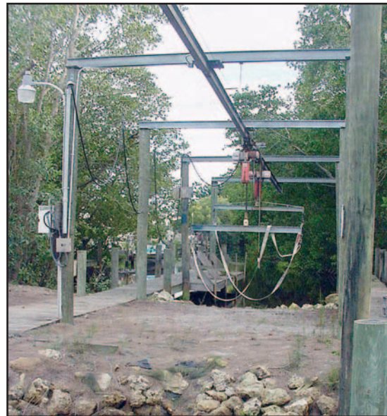
Boat lift at Flamingo Bay.
